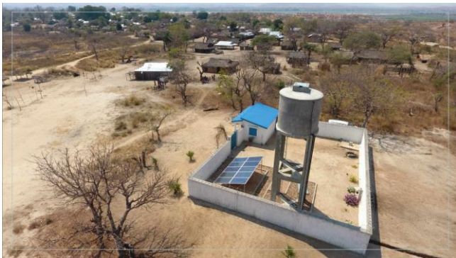
Water reservoir for a piped system in Madagascar, © charity: water
